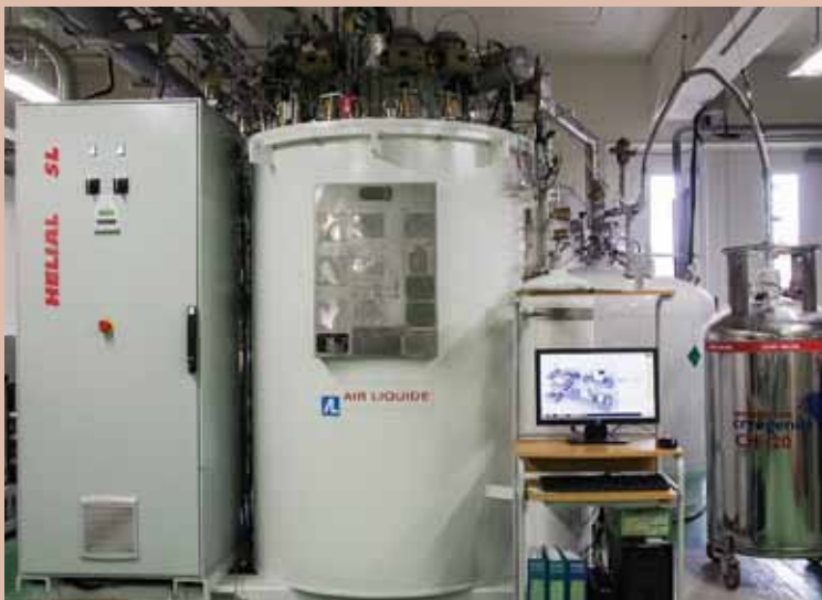
Fig. 1: Helium liquefier in CL
